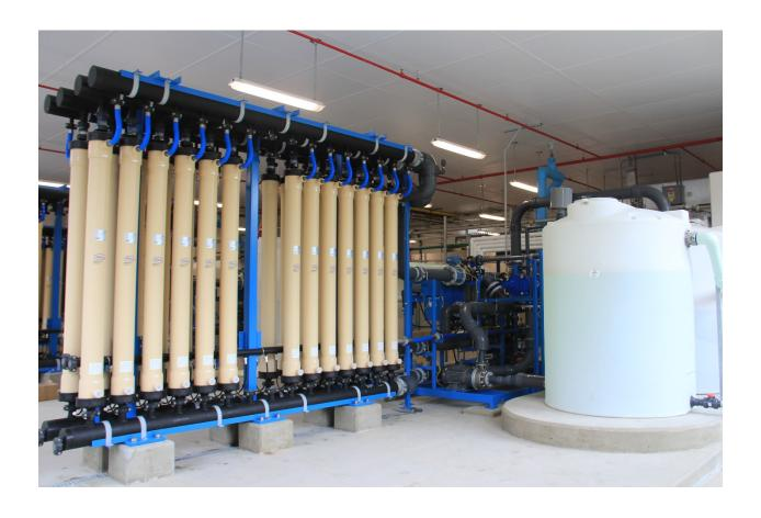
The Pall Microfiltration system is hard at work improving the water quality at the South Acton Water Treatment Plant.
